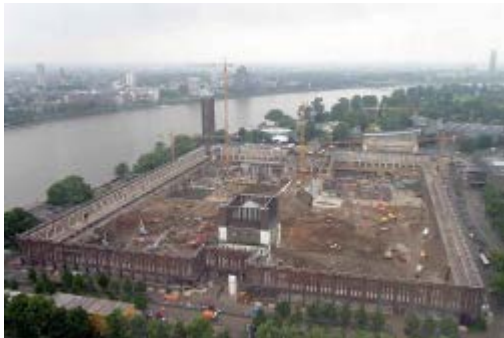
The historic fairground while it's renovation
