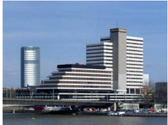
The old Lufthansa headquarter
